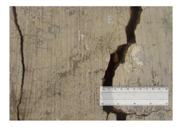
With "severe" wall cracks (15 to 25 mm wide) window and door frames may be distorted, floors slope noticeably, walls lean or bulge, some loss of bearing in beams, service pipes are probably disrupted and a gap of up to 20 mm between ceiling cornices and walls may appear.
