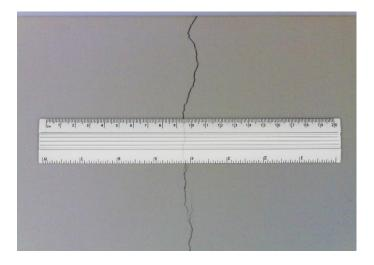
Settlement cracking is best repaired with a flexible crack filler. Because these cracks are "movement" cracks they are likely to reoccur. On the other hand, fine crazed cracking is a once-off defect and here the cracks can be filled and covered with paint or a suitable skimming material and are unlikely to reoccur.
